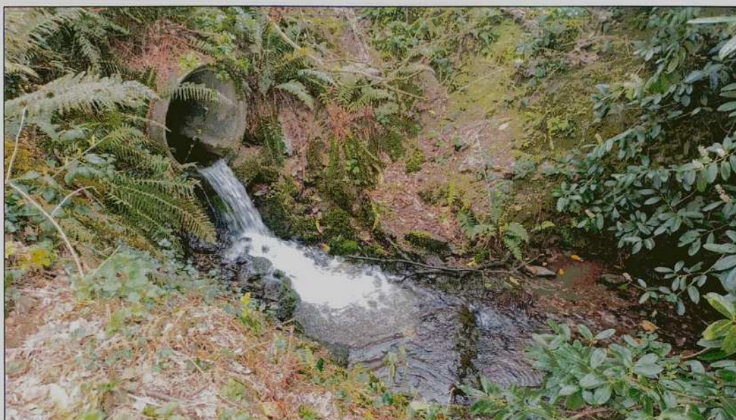
Concrete pipe culvert at the northern boundary of the site (i.e. the entrance point to the NE corner of the site)
