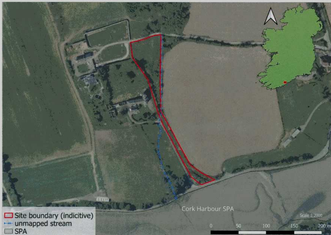
Figure 3. Overview of the proposed works area at Jamesbrook, East Ferry, Co. Cork, and position of stream.
